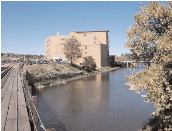
Buildings Encroaching on Water
