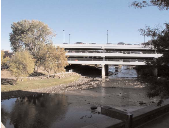
Parking Structure Over Waterway
