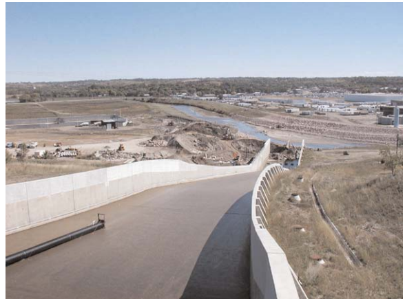
Large Water Spillway
