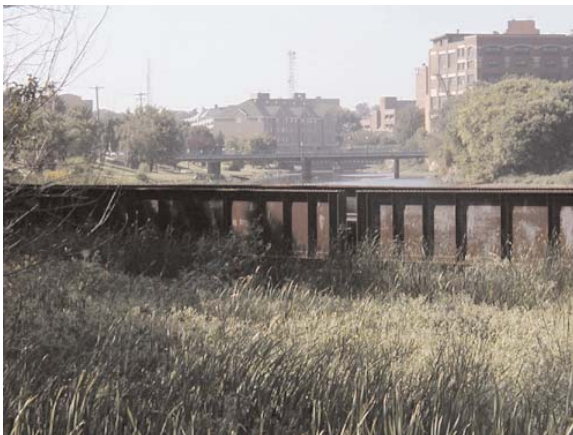
Railroad Bridge Relocation
