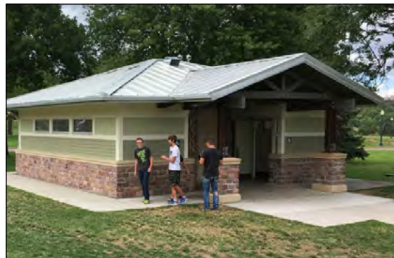
Falls Park Accessible Restrooms
