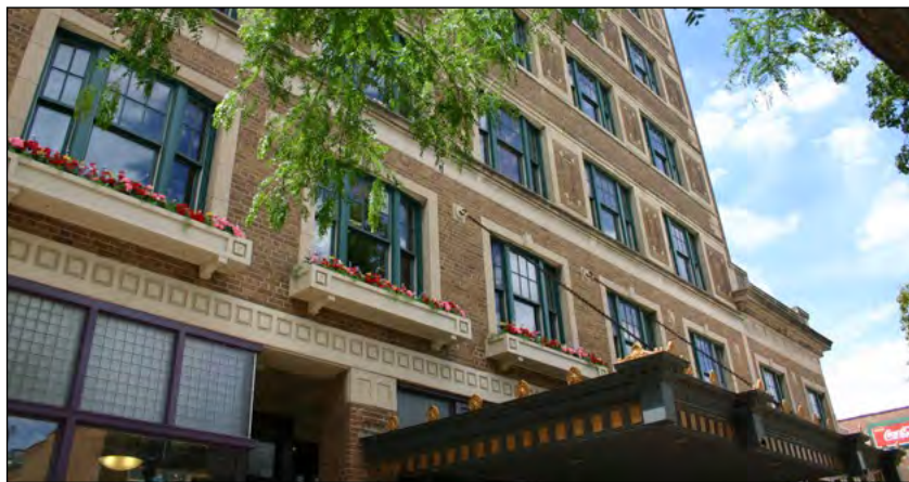
Architectural Enhancements, Downtown Carpenter Building
