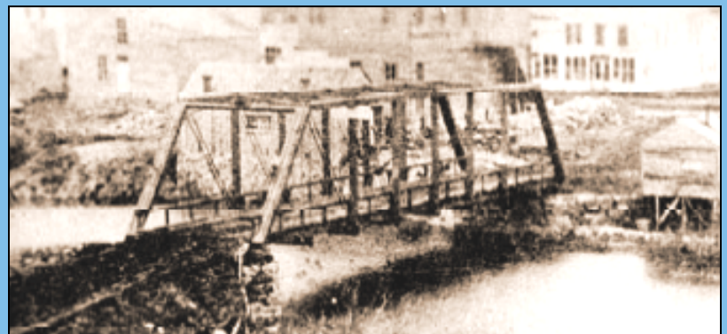
8th Street Bridge, 1876
