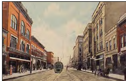
Trolley System, 1900s
